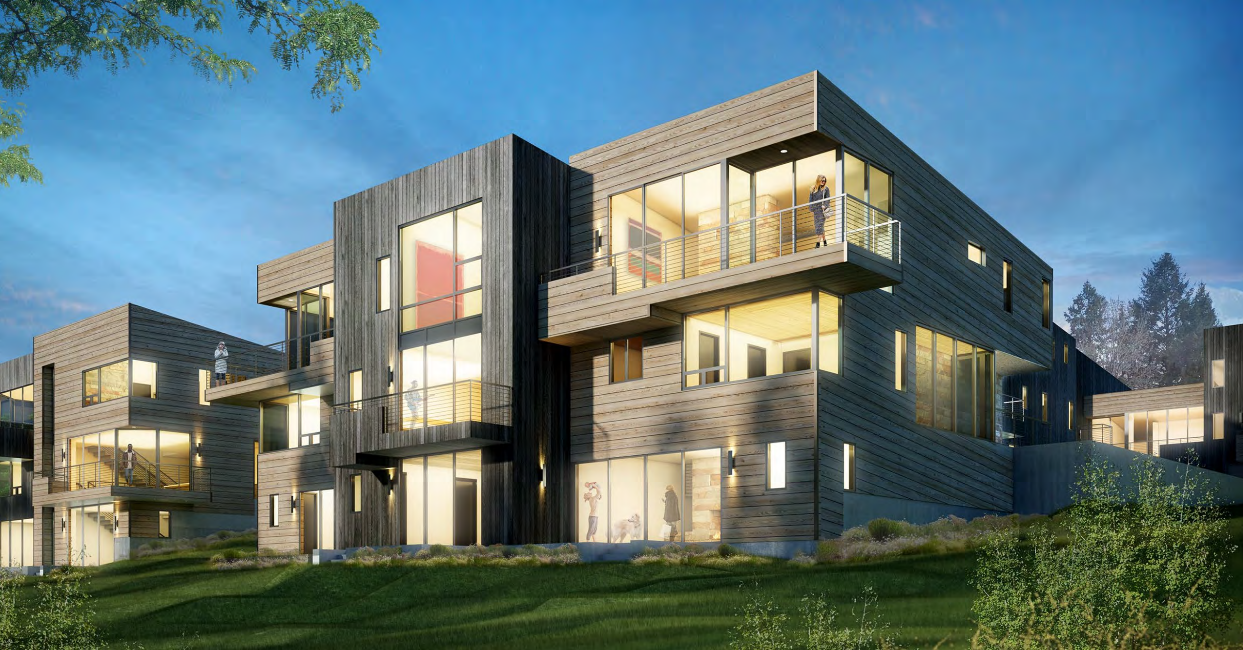
BUILDING 6: Looking Southeast
